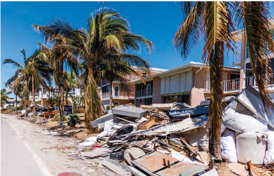
Damage caused by Hurricane Ian
